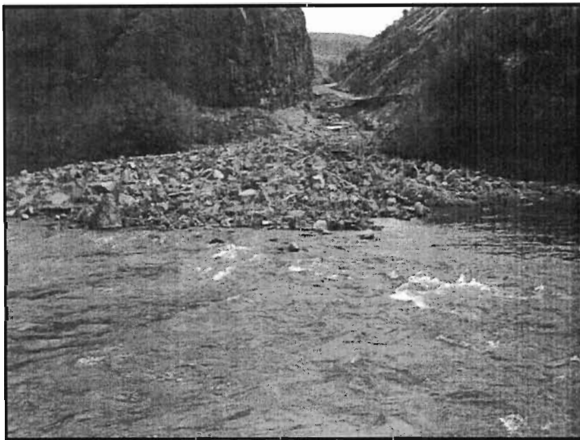
Wymer Cut along canyon highway is cut now. A significant amount of the road was washed away by the normally dry McPherson Creek which comes into the Yakima Canyon. All is not as bad as it looks, the slide created slow velocity summer rearing habitat for juvenile chinook. Photo courtesy Joe Jay Pinkham, III.
