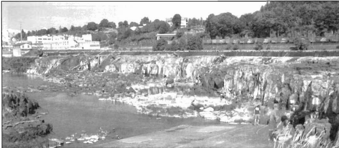
Above—At Willamette Falls river flows were cut off leaving adult steelhead and lamprey without adequate water to exist. The mill is to the left and expanse of the splash dam perimeter (darker portion) just below it. Far right—Tribal biologist looks down to check the damage.
